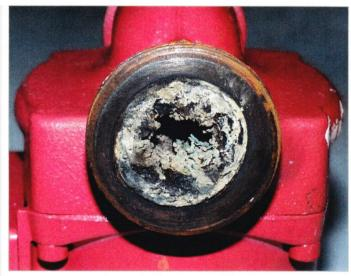
Figure 1: Magnetic corrosion debris in a circulator pump
